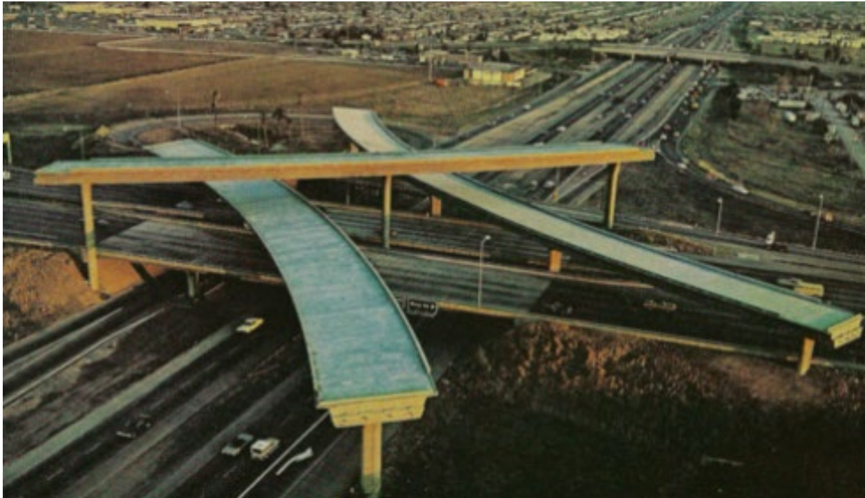
Figure ES-8. Unfinished US-101/I-280/I-680 Interchange, 1976
