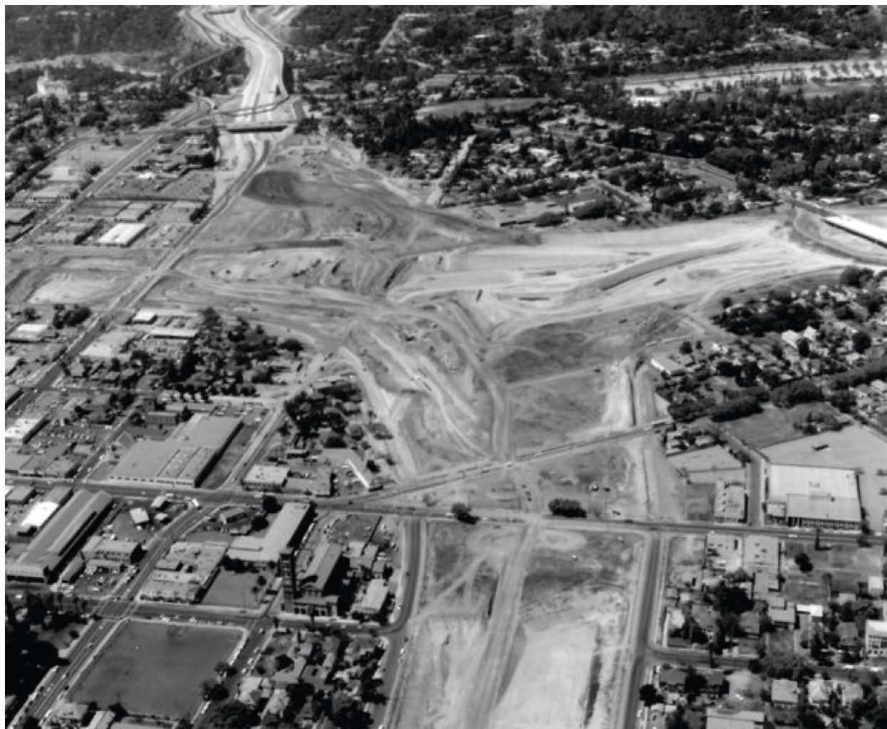
Figure 5-18. Cleared Land in Pasadena for Freeway Construction
