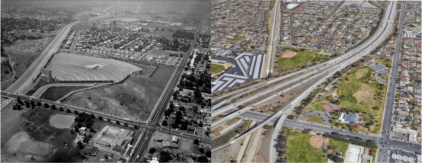
Figure 6-16. The Laurel Drive-in Theater before Freeway Construction, 1964, and the SR-118 Freeway on the Same Site Today
