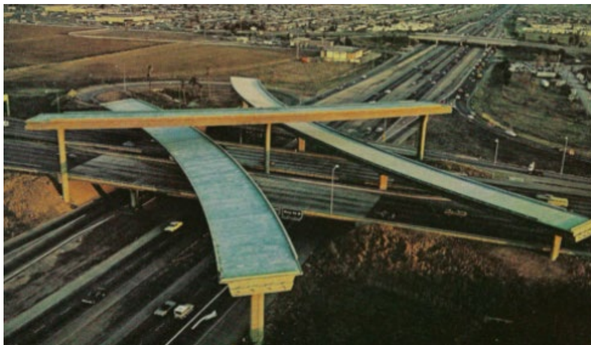
Figure 8-12. Unfinished US-101/I-280/I-680 Interchange, 1976
