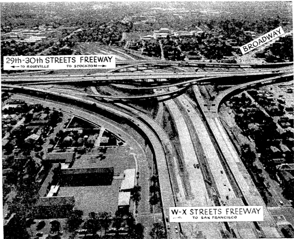
Figure 7-10. Incomplete Interchange of SR-99 (Left-right) and US-50 (Bottom)
