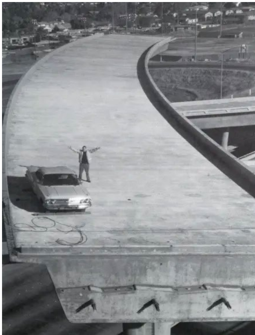
Figure 8-13. Joe Colla atop the Unfinished US-101/I-280/I-680 Interchange
